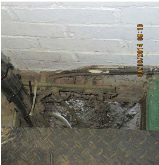
(a) An opening viewed from inside (Stone)
